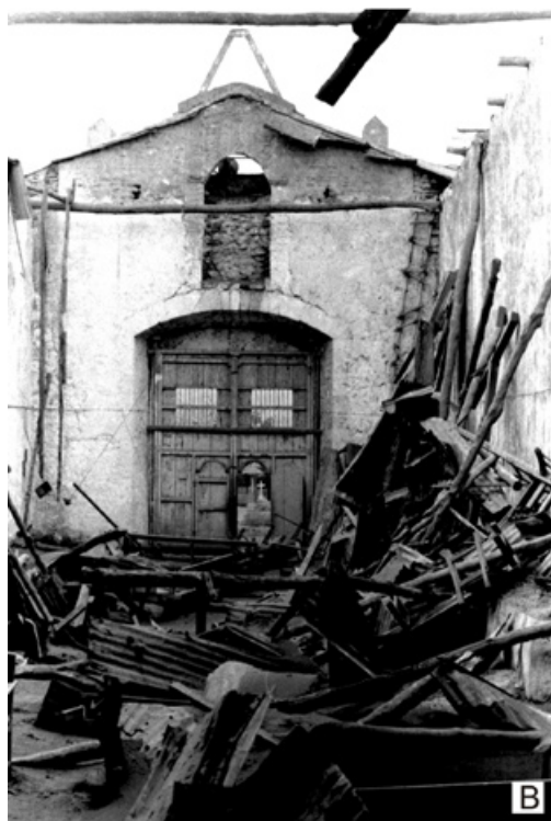
Fig. 4. A) Aerial view of the town of Naranjo, located south of El Chichón volcano (see Fig. 3). Notice the church with the collapsed roof. B) Close-up view of the church interior. Photographs by Rosa Plá Cortés taken in March 1982.
