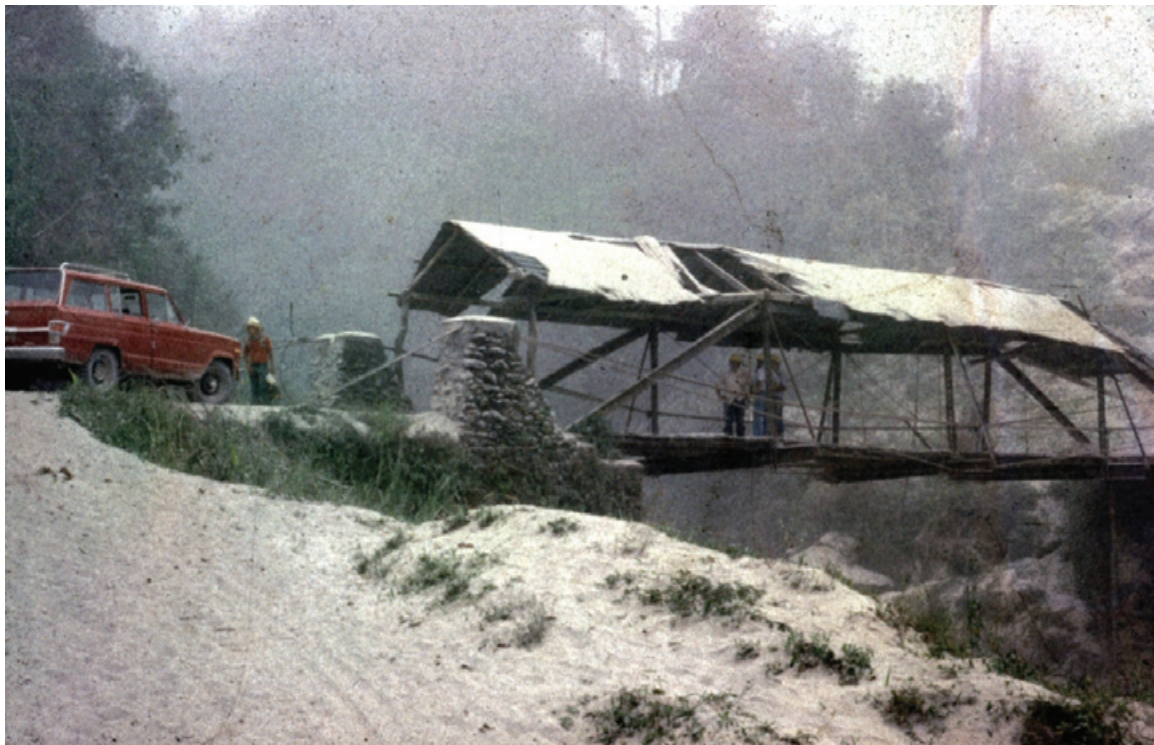
Fig. 3. Wooden bridge about 6 km from the volcano, partially destroyed by fall products of the March 28, 1982 El Chichón eruption (photo by S. De la Cruz-Reyna).
