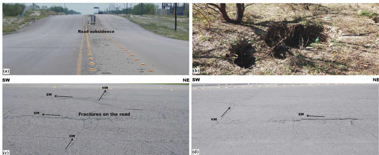
Figure 14. Sector 3. a) Image showing the subsidence of the road. b) Image of a sinkhole next to the road. c) and d) Images of fractures on the road surface in Profile P1. Reference points for the photographs shown in c) and d) are indicated as F1 and F2 in Figure 7, respectively.
