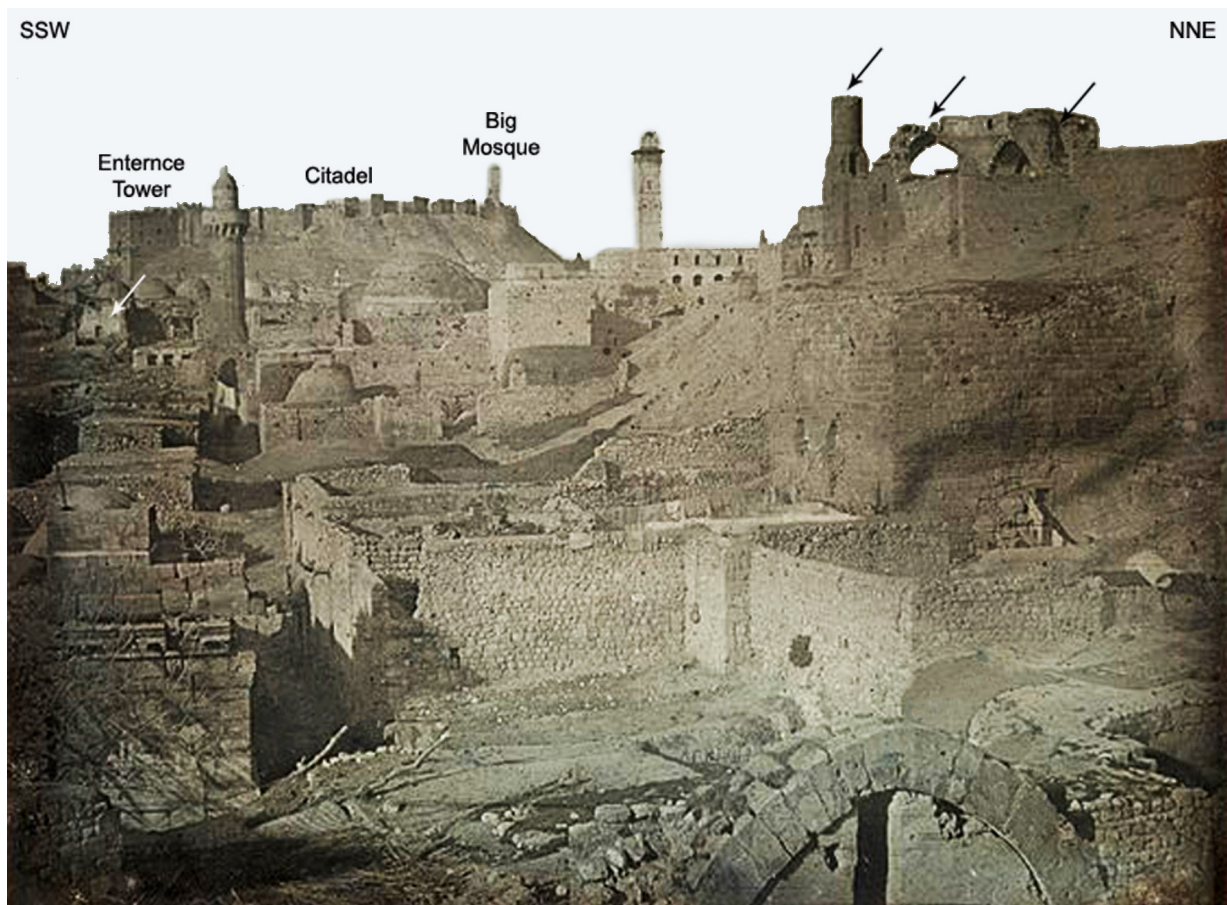
Figure 5. The earliest known photograph of Aleppo taken in 1844 by the French photographer Joseph-Philibert Girault de Prangey (1804-1892) showing the miserable condition of the city due to the 1822 earthquake (black arrows). Source: Metropolitan Museum of Art at: https://www.metmuseum.org/art/collection/search/726483
